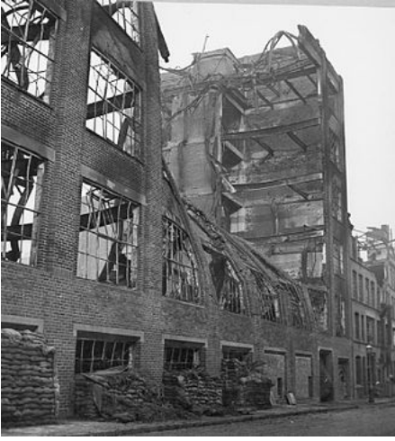
A ruined factory building.
